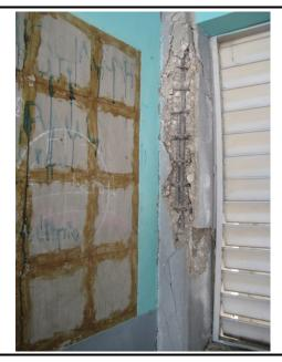
Extensive spalling of first-story column. (NEEShub, 2010)
