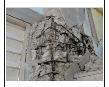
Close-up of shear damage in first-story column. (NEEShub, 2010)
