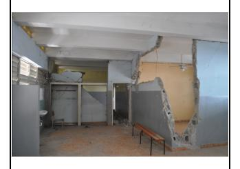
Severe damage to nonstructural URM walls. (NEEShub, 2010)
