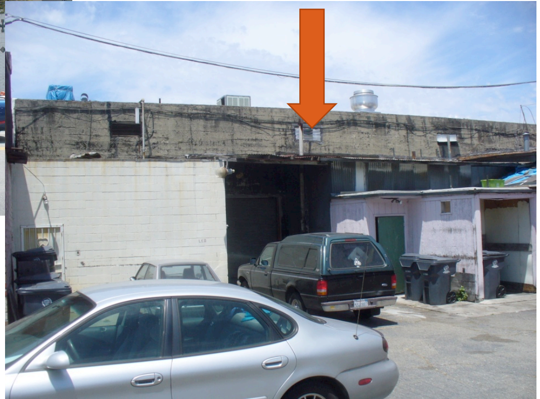
Concrete in the back
