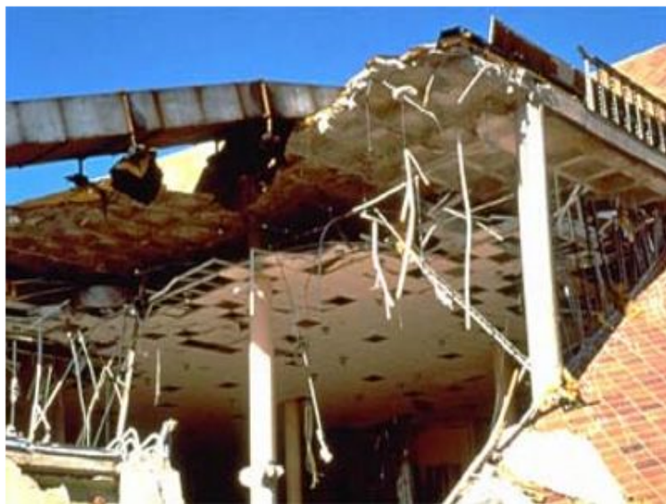
Northridge 1994 shear failure between waffle slabs and columns
